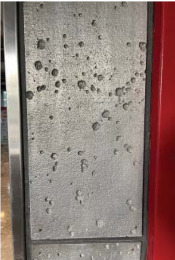
Below: A closeup of one of the lunar finish concrete panels. This one is painted in a metallic silver.
