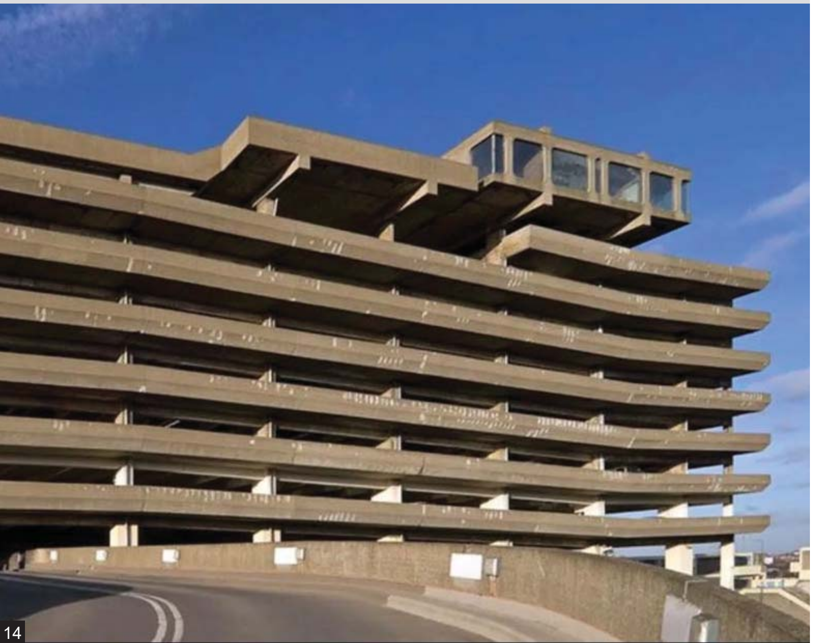
14. Trinity Car Park, Gateshead, England, UK 1971. Note the application of chamfering on the lower edge of the horizontal blocks.
