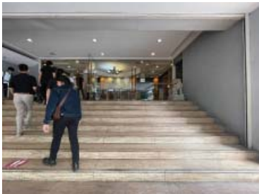
Above: Imported natural stone-clad stairway to the main lobby--noticably different from Locsin's preference for pebble-dash for entry stairways. Locsin would also typically make use of shadow lines to create a series of seemingly levitating steps.
